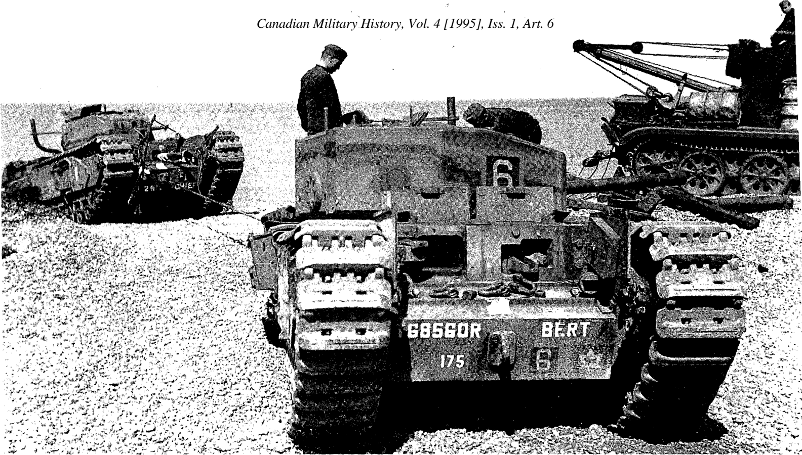
BERT was immobilized on the promenade when shell fire broke its left track. After the battle it was repaired by German engineers and is seen here towing CHIEF off the beach. Bundesarchiv 291/1242-2A
